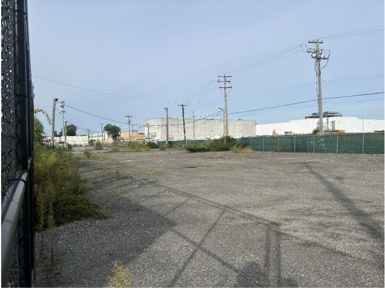
Photograph #1. View of the Commercial Avenue Terminal parcel. Note light oil staining. Photo taken September 30, 2025 by PS&S.
