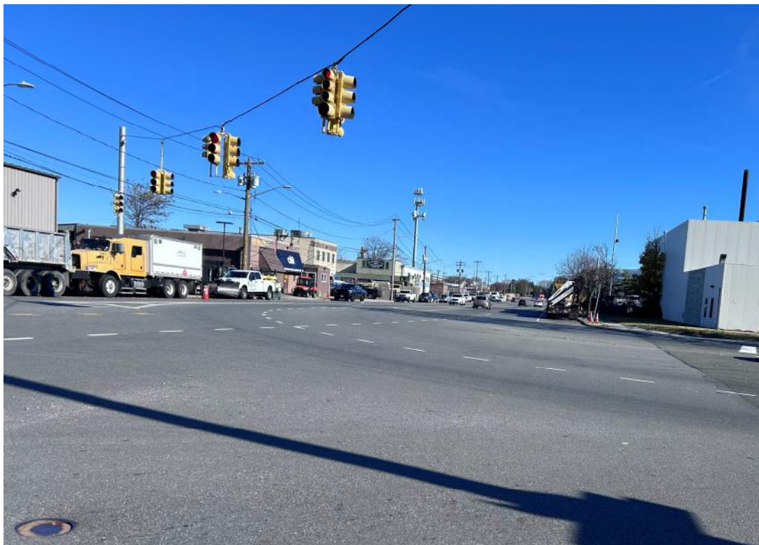
Photograph 2: View of the western freeze pit work area near the intersection of Commercial Avenue and Oak Street.
