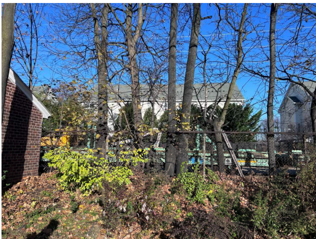
Photograph # 8: View near the eastern freeze pit work area within LIRR property facing north.
